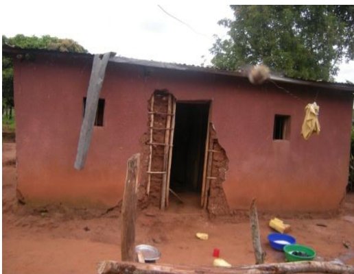
A House before repair
