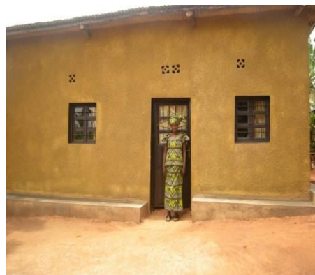
A House after repair
