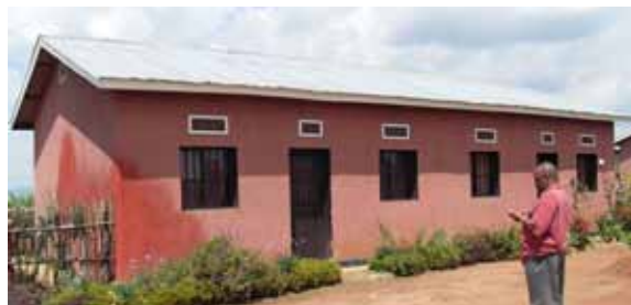
SURF Coordinator, Gabo Wilson, at a new home constructed for survivors in Kamonyi, October 2009 © SURF
